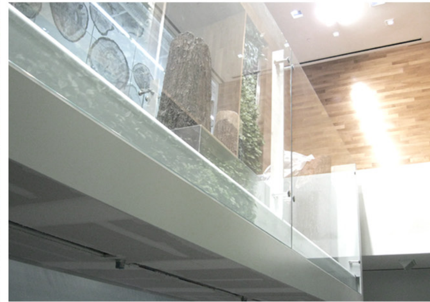
20 foot x 5 foot planter above conference table in FVG. Contains full sized red-wood trunks and other riparian plantings. False walls give the impression of a deeper planting bed.
