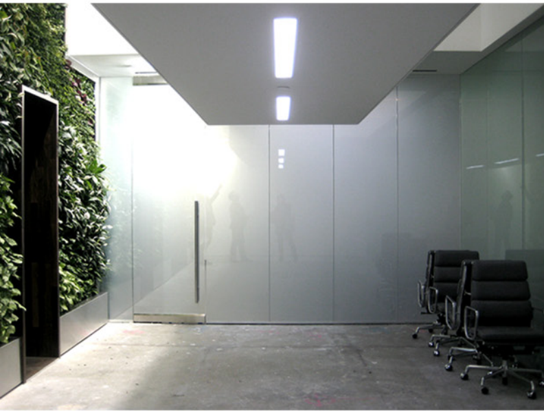
Privacy in conference spaces provided by smart glass panels
