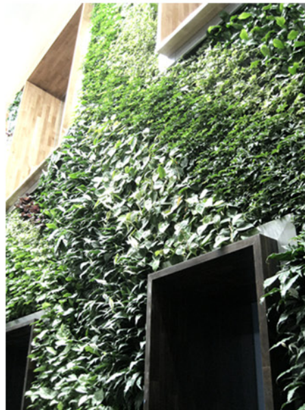
2-story green wall
